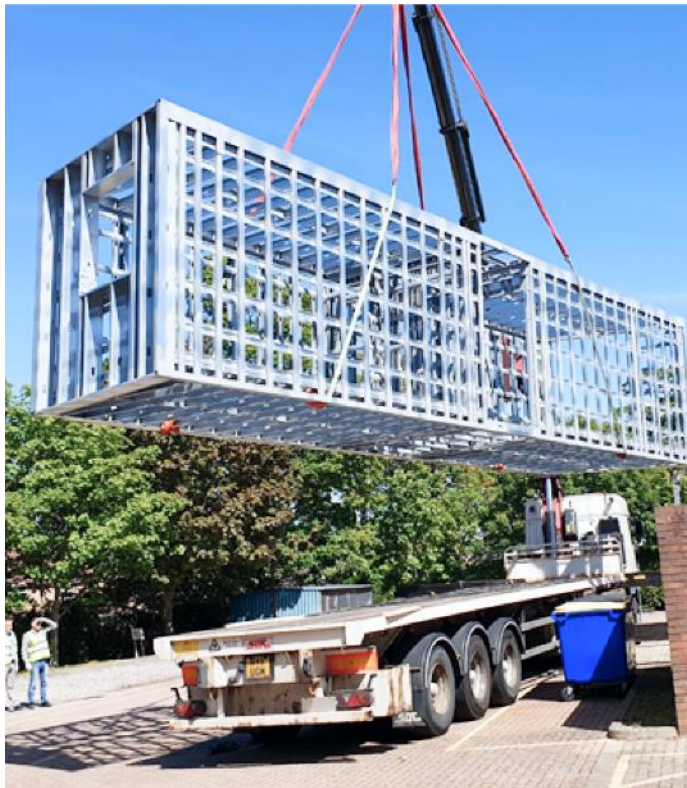
METAL FRAME PRODUCTION
