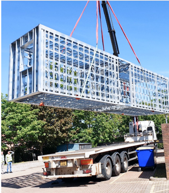
METAL FRAME PRODUCTION
