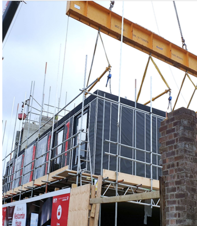
FINISHED MODULE INSTALLATION
