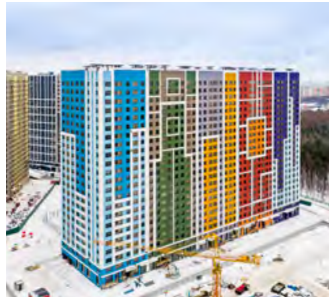
ETALON CITY BUILDING 2, DELIVERED IN 2016
